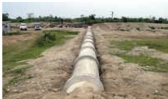
3rd Party Monitoring of Hume Pipe Irrigation Conveyance System constructed under SPA 2009-10
