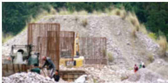
Third Party Monitoring of Construction of permanent bridge over river Sisiri on Dambuk Paglam road (RIDF-XII)
