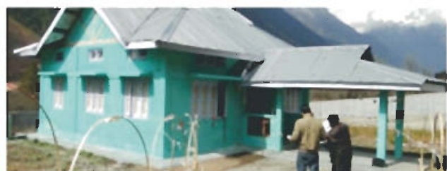
SPA project in Arunachal Pradesh
