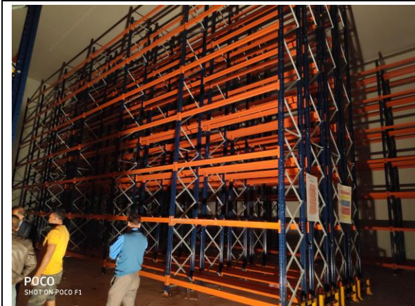
Inside view of Kharupetia Cold Storage
