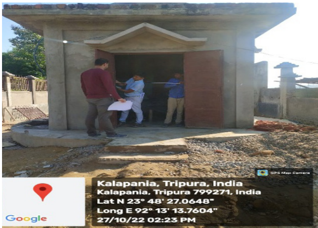
Inspection of pump house under JJM Tripura
