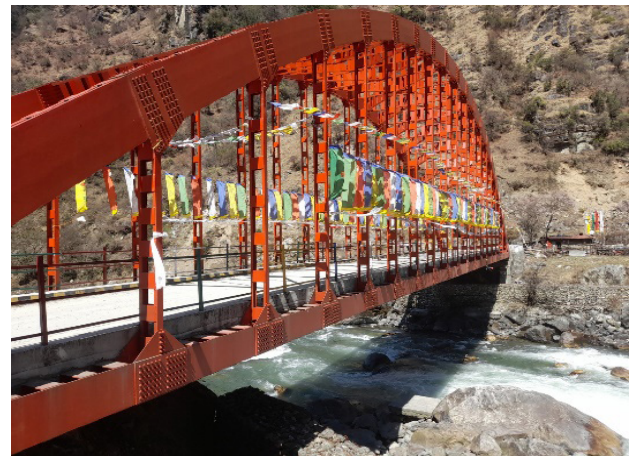
Monitoring of bridge executed under CSS scheme in Arunachal Pradesh
